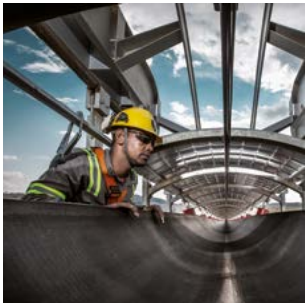
Installing the flying belt in Barroso, Brazil
